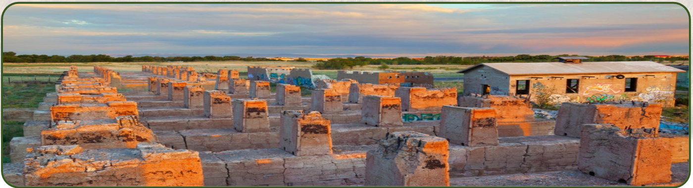
Background: current construction and business development in the rehabilitated area (looking east). Above: Early view of the Yttrium Plant (looking north) prior to cleanup.
