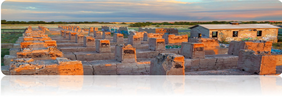
Early view of the Yttrium Plant (looking north)
